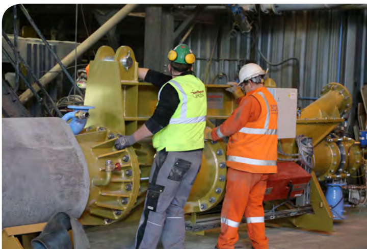
Figure 4. Hope and Unitherm engineers during installation.
