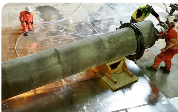
Figure 2. Air film pads for transportation of burner.
