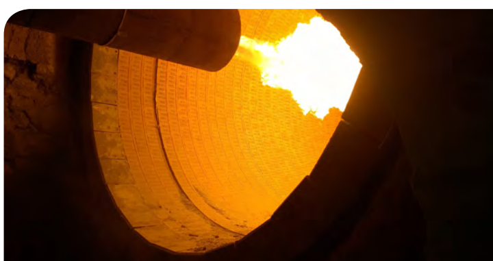
Figure 5. Oil established. Successful commissioning of the first Unitherm burner at Hope.
