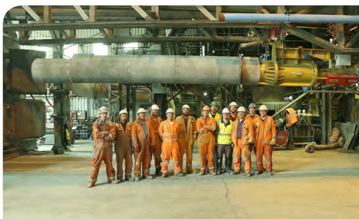
Figure 3. Hope and Unitherm engineering team during installation.
