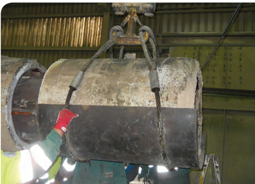
Figure 5. Removing the front jacket tube.
